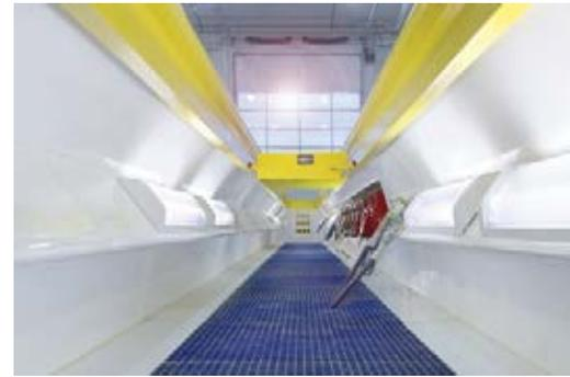
Floor surfaces are made of fiberglass grating for a non-slip surface and to allow spilled oil and other fluids to drain to an integral sump. The interior is bright white with an easy-to-clean gel-coat finish combined with built-in lighting to make chassis inspections fast and efficient.
